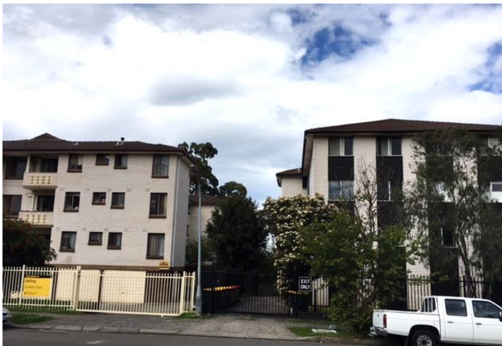
Figure 6 Residential flat buildings located opposite (east) of the site
