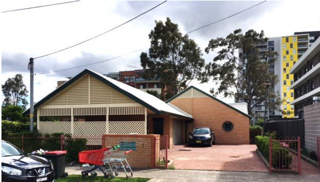
Figure 5 No. 7 Goulburn Street Warwick Farm to the north of the site
