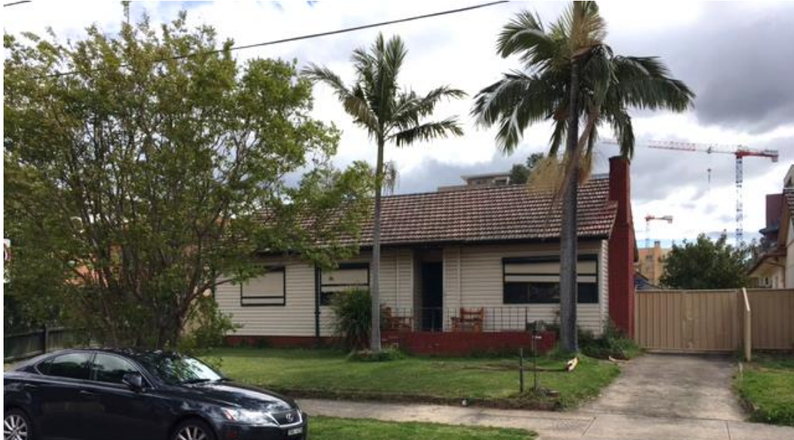
Figure 4 No.13 Goulburn Street, Warwick Farm
